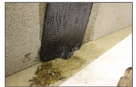
Twist carbon fiber and insert into hole
