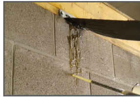
01: Lift carbon fiber strap & apply epoxy to wall
