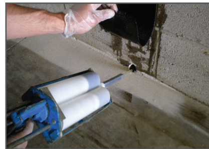
Apply epoxy to hole
