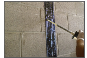
03: Apply carbon fiber strap & coat with epoxy
