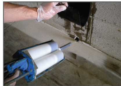
Apply epoxy to hole
