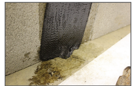
Twist carbon fiber and insert into hole
