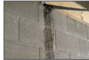
02: Spread epoxy on foundation wall
